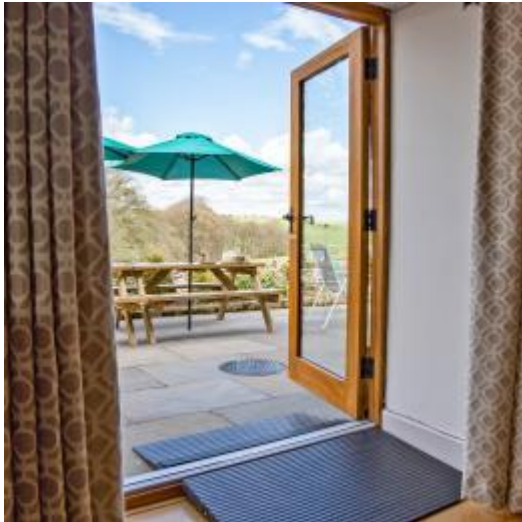
Ramp to patio
